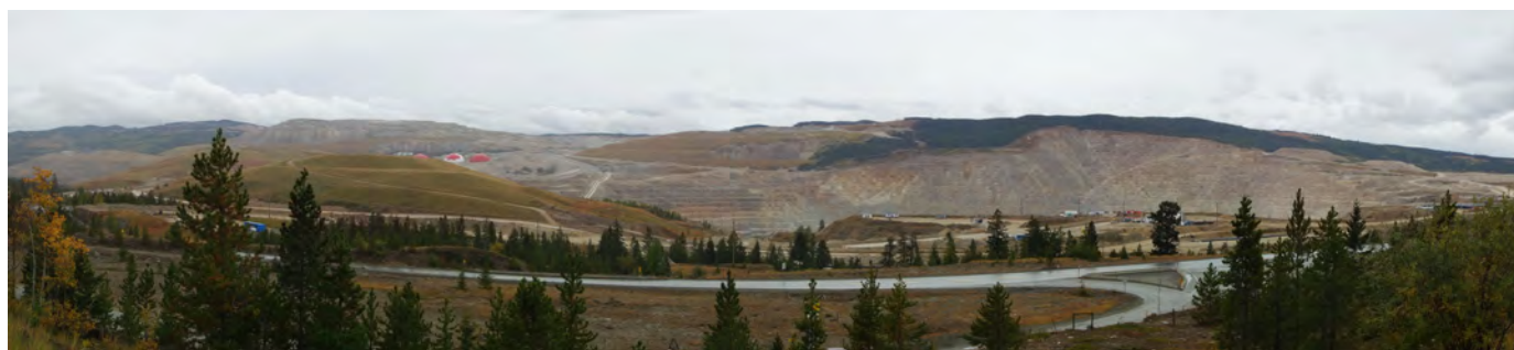
Fig. 2. Highland Valley Copper copper-molybdenum mine. The Valley pit looking southwest from a viewpoint off Highway 97C. Ore is currently mined from the Valley pit and Lornex pit to the south. The past-producing Bethlehem pit (to the east, out of view) is a proposed expansion area.
