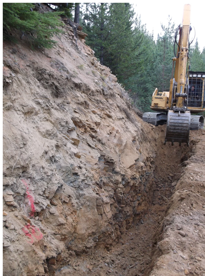
Fig. 8. BC Sugar graphite project. Lithium Corporation is studying results of 2015 trenching (shown here). Graphite occurs as thin seams in metasedimentary rock of the Shuswap metamorphic complex, east of Mabel Lake (Image courtesy of Lithium Corp.).
