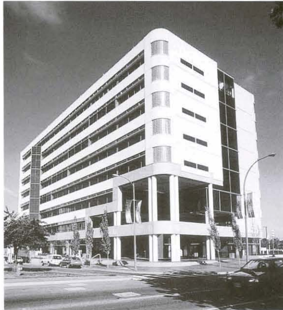
The Jack Davis Building displays two types of granite: one for the wall facings, and a second as floor tiles.
