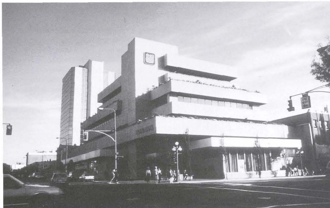
The facing of the Royal Bank is made of precast concrete blocks with a Beaverdell granite aggregate.
