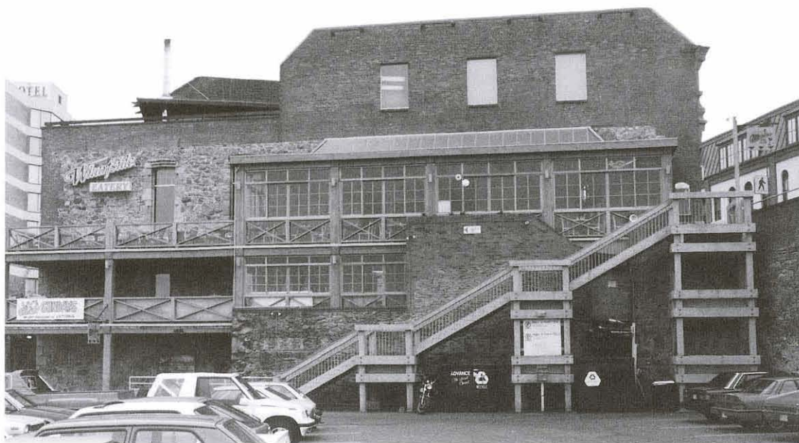
Mortared fieldstone wall below Wharfside Eatery.
