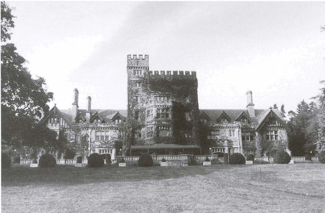
Royal Roads was built with various sandstones and with granite that was most likely quarried on site.
