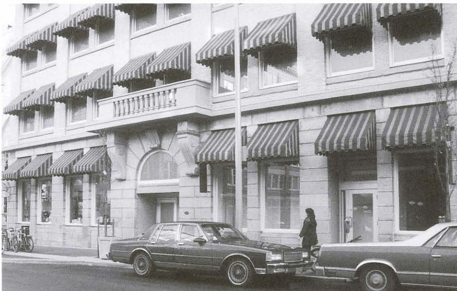
Sandstone forms the base of this portion of the preserved heritage facades – Eaton Centre.
